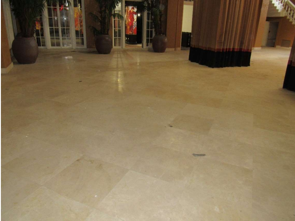
Photo #33 Gulfstream Hotel Building 1 Lake Ave, Lake Worth, FL 33460 Close-up of tile flooring in lobby (7/10/2020)
