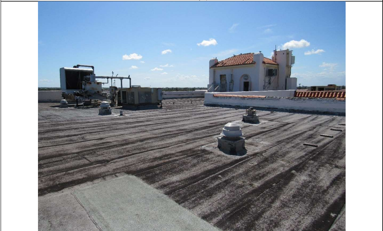
Photo #75 Gulfstream Hotel Building 1 Lake Ave, Lake Worth, FL 33460 Rooftop (3/12/2020)
