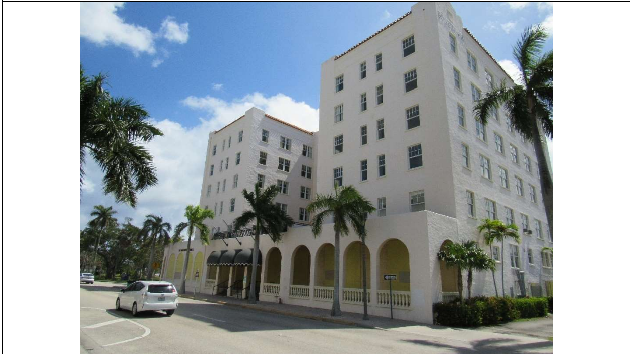
Photo #4 Gulfstream Hotel Building 1 Lake Ave, Lake Worth, FL 33460 View of NW corner (3/12/2020)
