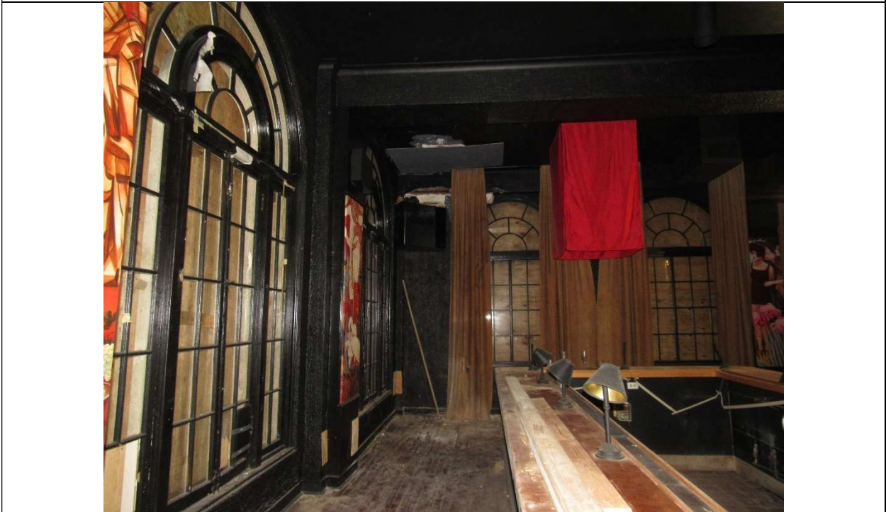
Photo #28 Gulfstream hotel Building 1 Lake Ave, Lake Worth, FL 33460 East wing facing N (7/10/2020)
