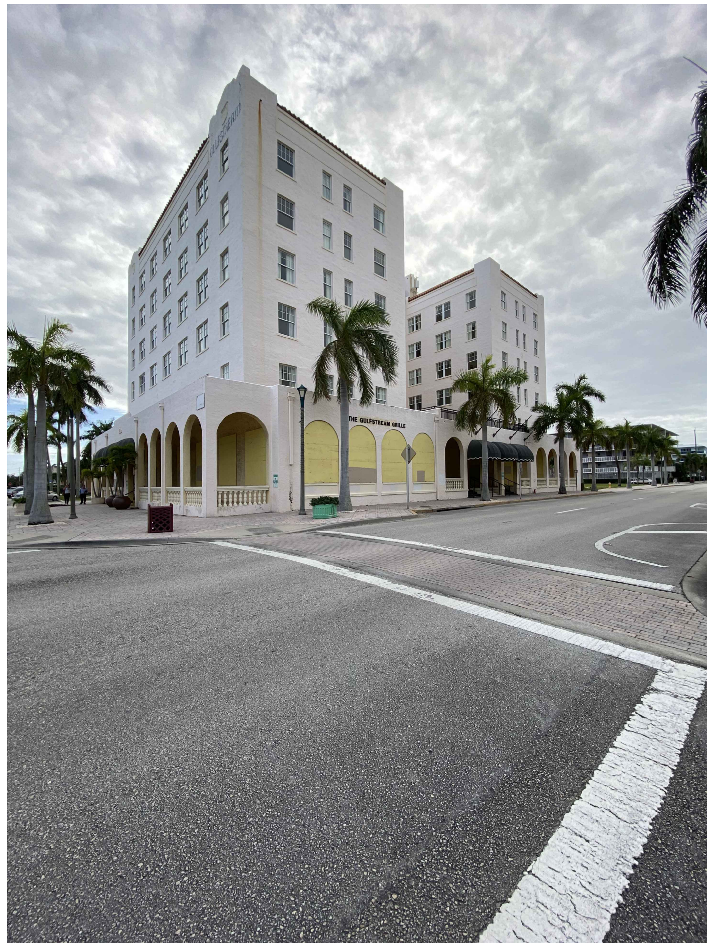
EXISTING BUILDING LOOKING SOUTHWEST
