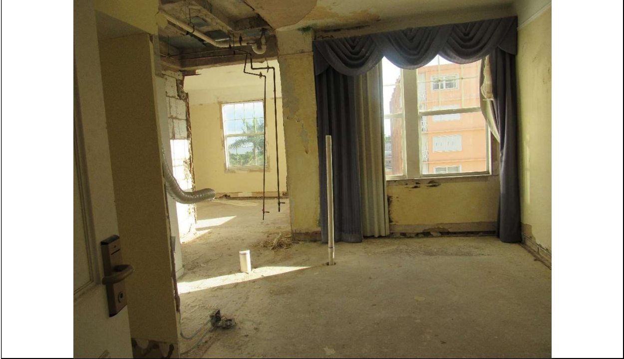
Photo #58 Gulfstream Hotel Building 1 Lake Ave, Lake Worth, FL 33460 Fourth floor room (7/10/2020)
