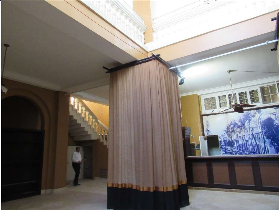
Photo #16 Gulfstream Hotel Building 1 Lake Ave, Lake Worth, FL 33460 Lobby area facing SE (11/7/2019)
