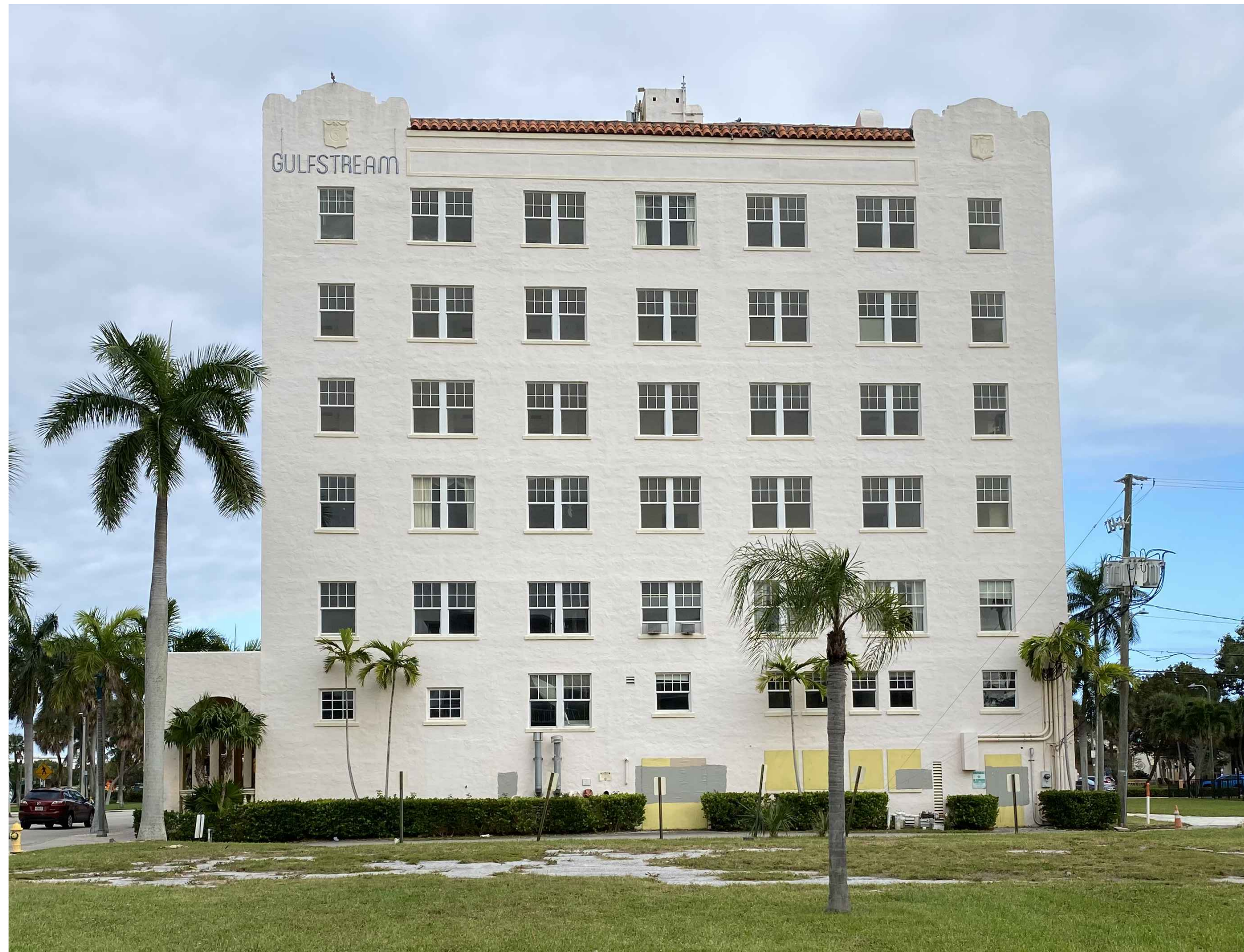
EXISTING BUILDING LOOKING EAST
