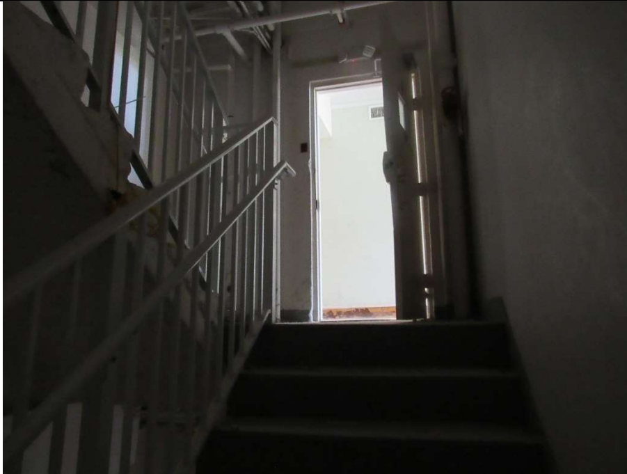
Photo #51 Gulfstream Hotel Building 1 Lake Ave, Lake Worth, FL 33460 Stairwell to third floor (7/10/2020)
