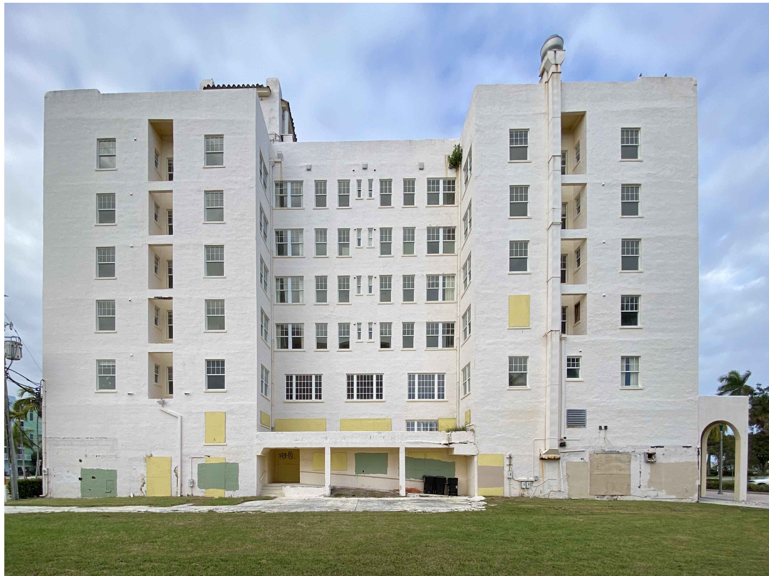
EXISTING BUILDING LOOKING NORTH
