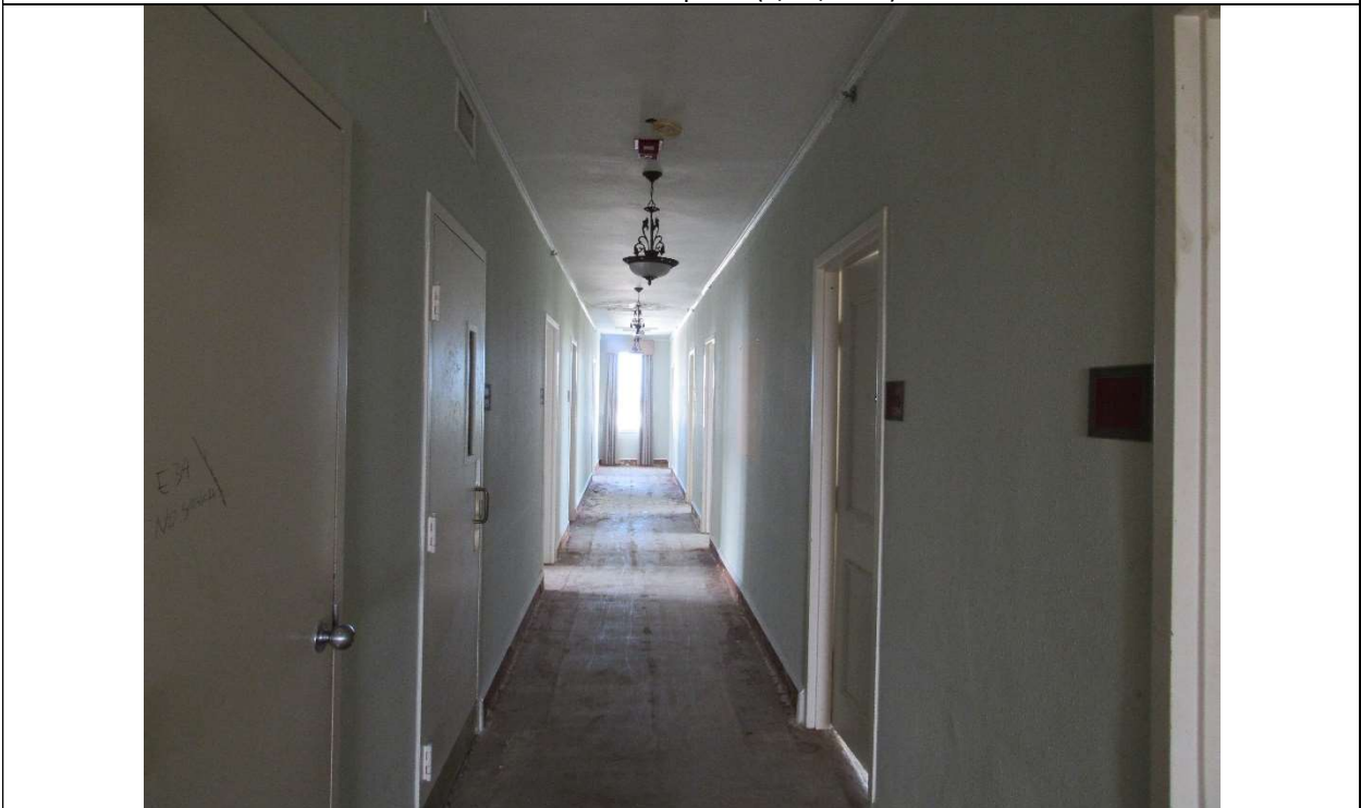
Photo #73 Gulfstream Hotel Building 1 Lake Ave, Lake Worth, FL 33460 North view of first floor interior windows (7/10/2020)
