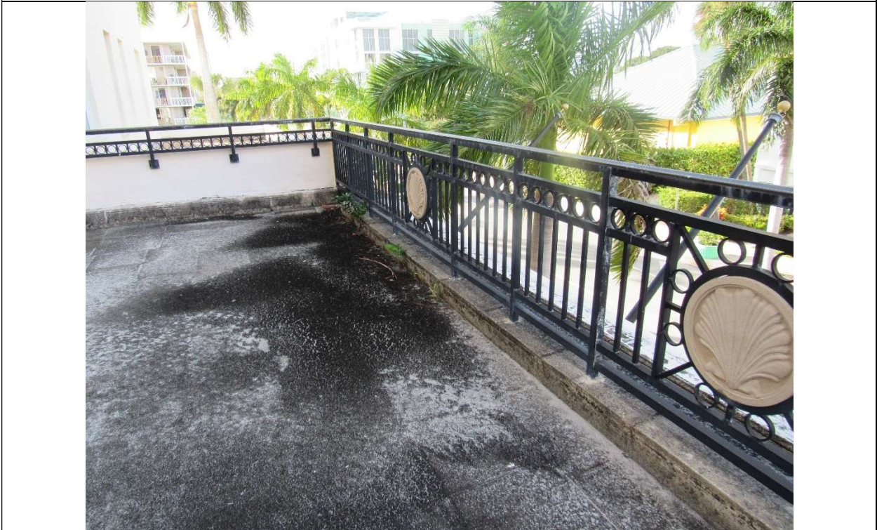
Photo #47 Gulfstream Hotel Building 1 Lake Ave, Lake Worth, FL 33460 Exterior space N elevation (7/10/2020)
