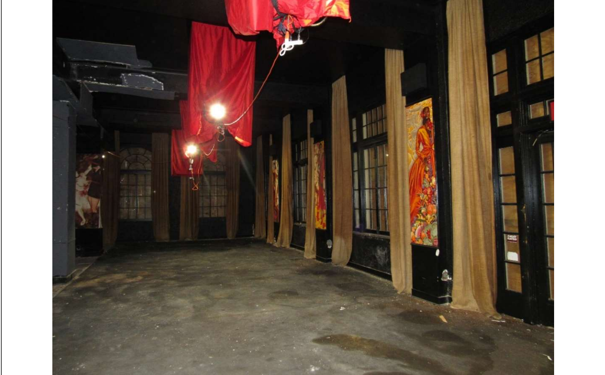
Photo #31 Gulfstream Hotel Building 1 Lake Ave, Lake Worth, FL 33460 East wing facing S (11/7/2019)
