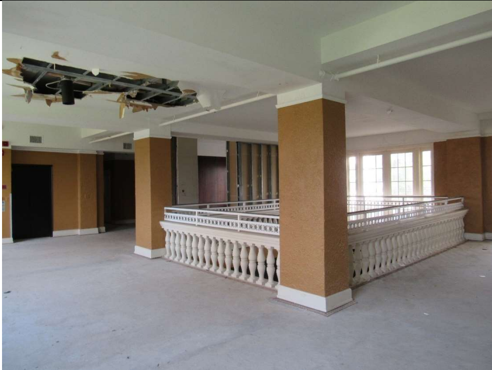
Photo #41 Gulfstream Hotel Building 1 Lake Ave, Lake Worth, FL 33460 Mezzanine Area (7/10/2020)
