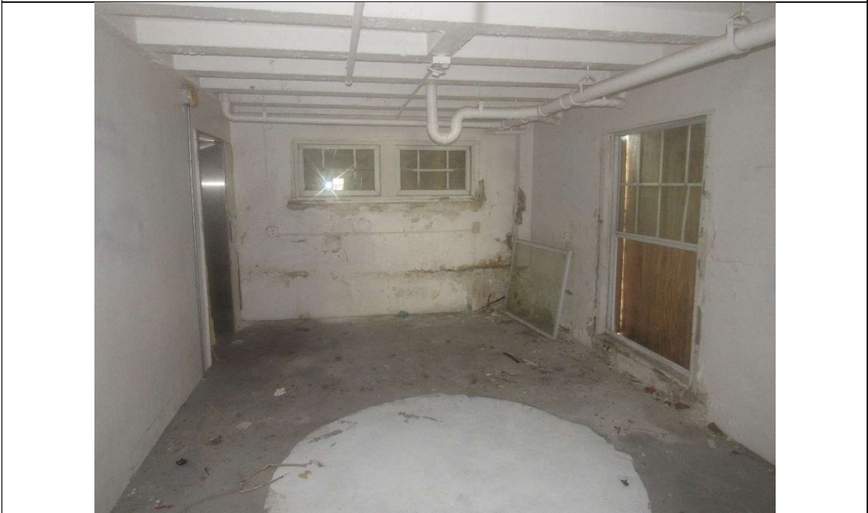
Photo #37 Gulfstream Hotel Building 1 Lake Ave, Lake Worth, FL 33460 Mechanical elevator lobby (7/10/2020)
