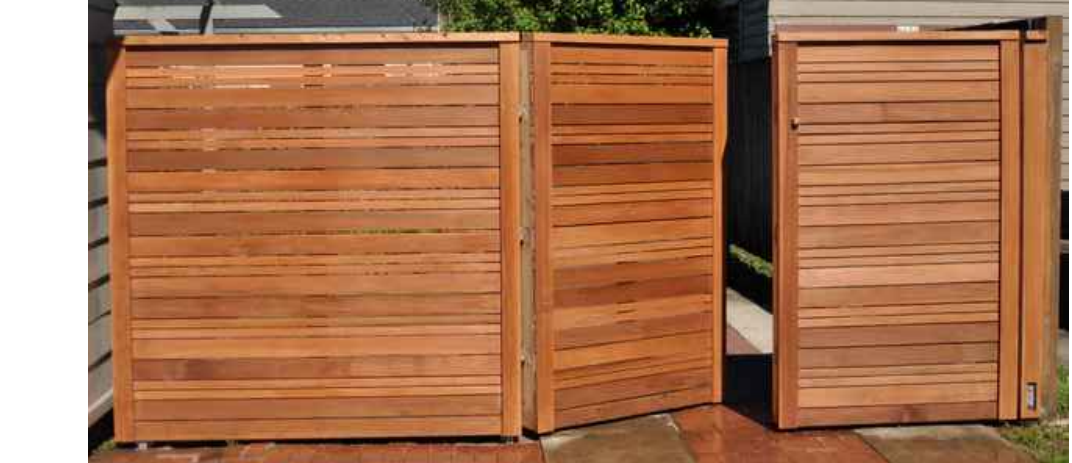
Typical 6' Opaque Screening Fence
