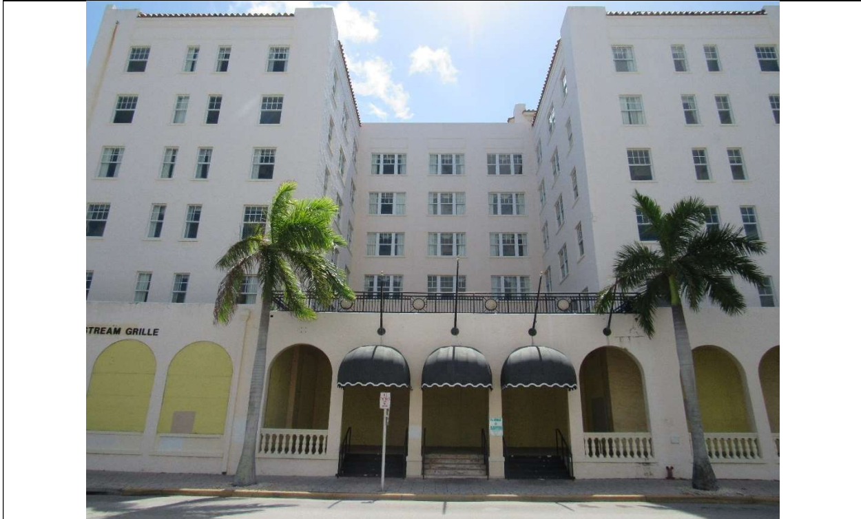
Photo #3 Gulfstream Hotel Building 1 Lake Ave, Lake Worth, FL 33460 View of entrance N Elevation (3/12/2020)
