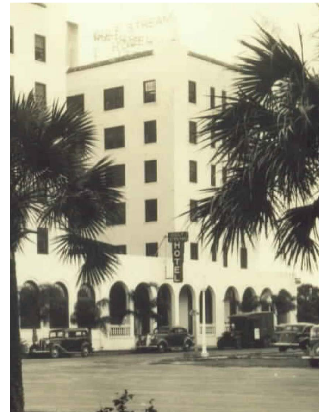
ORIGINAL SIGNAGE @ NORTH ELEVATION
