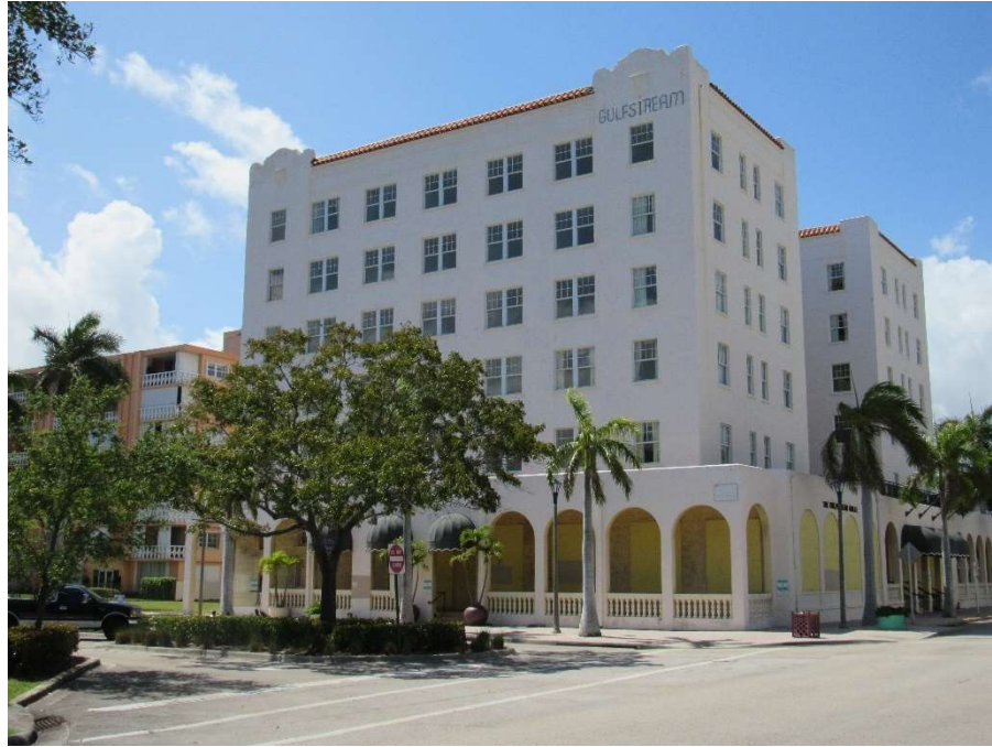
Photo #1 Gulfstream Hotel Building 1 Lake Ave, Lake Worth, FL 33460 View of NE Corner of Building (3/12/2020)
