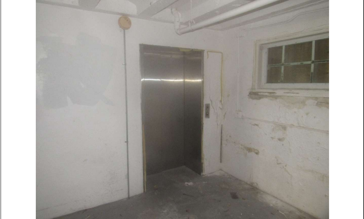
Photo #36 Gulfstream Hotel Building 1 Lake Ave, Lake Worth, FL 33460 Existing elevator (7/10/2020)
